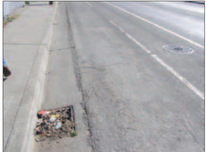
View of existing blocked storm drain inlet
