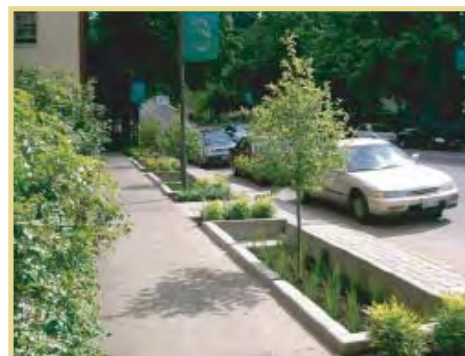
Planter boxes collect stormwater runoff, helping to irrigate landscaping.
