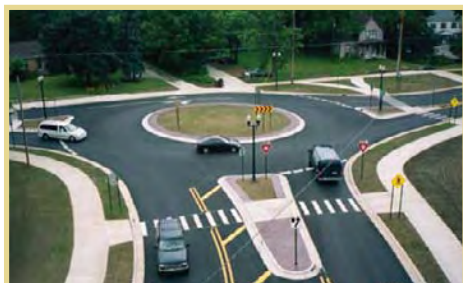
Roundabouts are raised islands that control competing vehicular movements.
