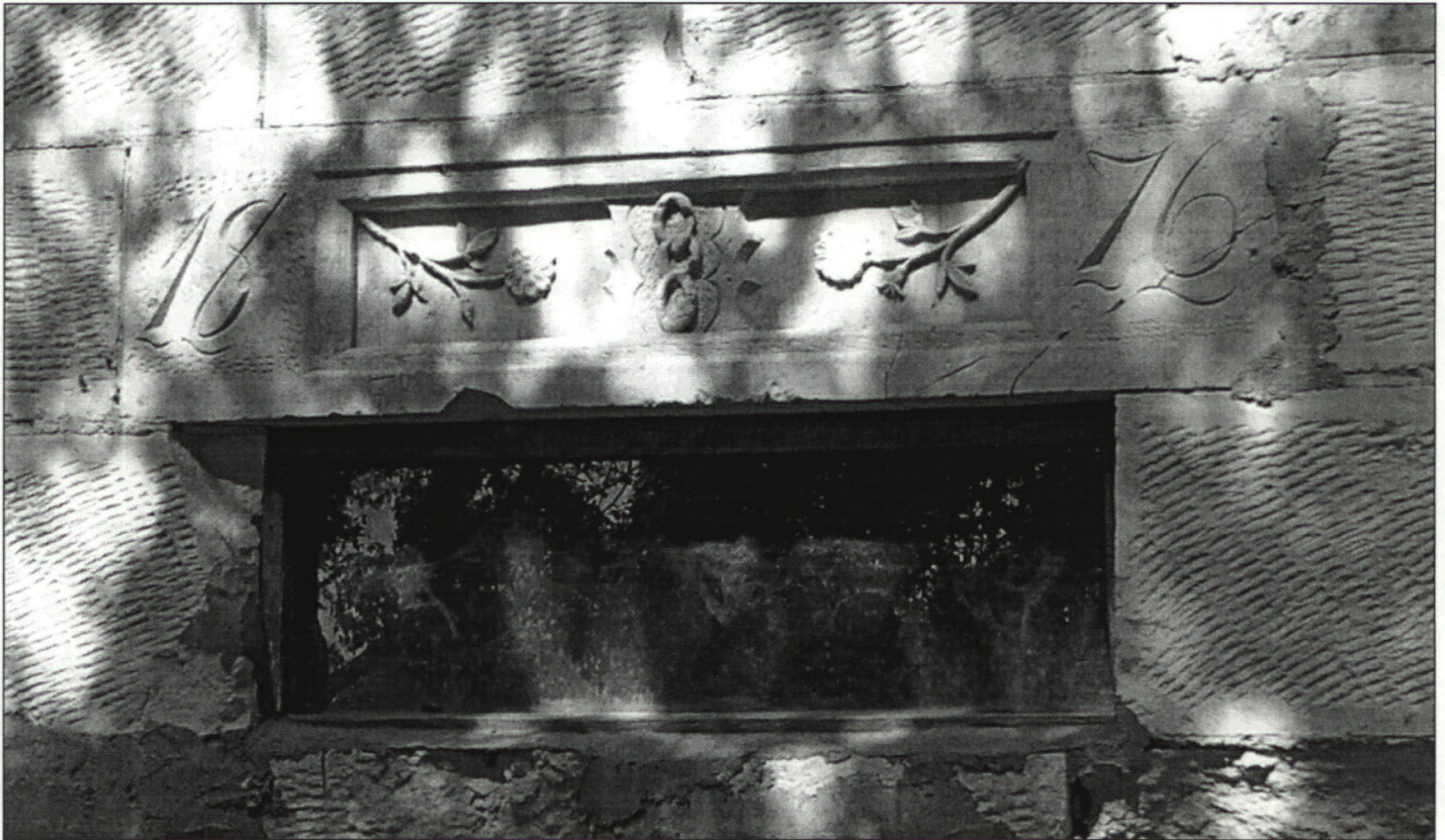
Lintel Detail (1876 carved on either side of floral design), Post Office
